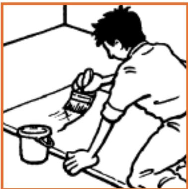
b) Make sure floor is clean and free from all loose material. NO MORE PLY boards must be primed both sides with one coat of SBR primer (one part SBR to three parts water). For best results lay NO MORE PLY on single part flexible rapid set adhesive ensuring joints are staggered.
