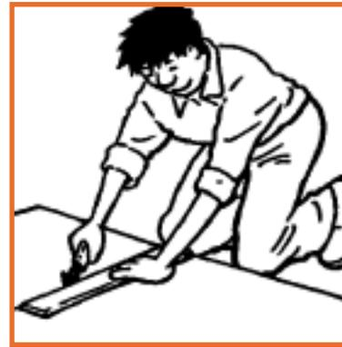
c) For straight cuts score with the NO MORE PLY Scoring Knife and snap. For curves and shapes use a jigsaw or nibble round pipes with tile nippers.
