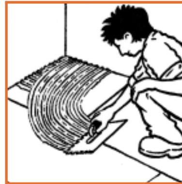
d) When floor is covered with NO MORE PLY, allow adhesive to set – see adhesive manufacturer's instructions on setting time. Sweep floor clean and you are ready for tiling.
